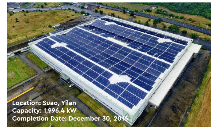
Photovoltaic System on the Roof of Pihsiang Machinery
