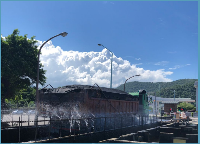
Port of Suao combines vehicle scales with car washing stations to make pollution control more efficient and effective.
