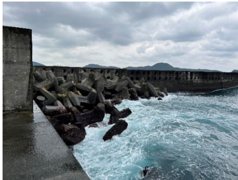
Reinforcement and Placement of Wave Breakers on South Breakwater
