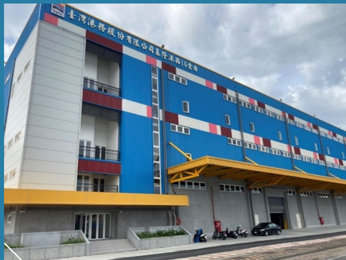
Keelung Port's West 16 Warehouse (Green Building)
