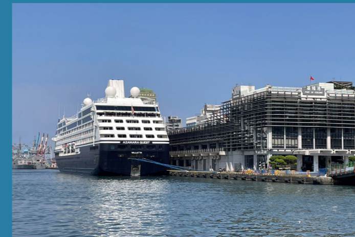
Lightweight aluminum grille facade of the Travel Center building
