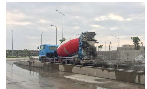
Carwash facilities clean vehicles exiting construction sites to prevent dust emissions from vehicles.
