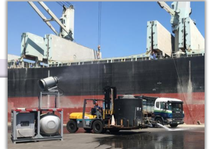
For the details of current onsite pollution preventive actions, there must be at least one water spray for every grabber to minimize dust. Furthermore, grabber shall not release the cargo until it reaches the bottom of the truck.
