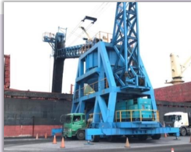
Port of Suao will continue to ensure stevedoring companies apply pollution preventive devices properly (dust net, water spray, etc.)
