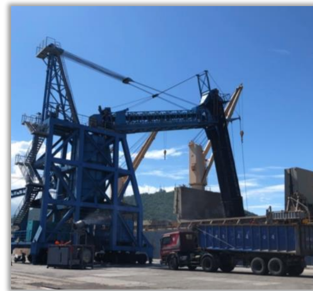
Port of Suao uses automatic coal unloading machine to reduce one of its main air pollution sources.
