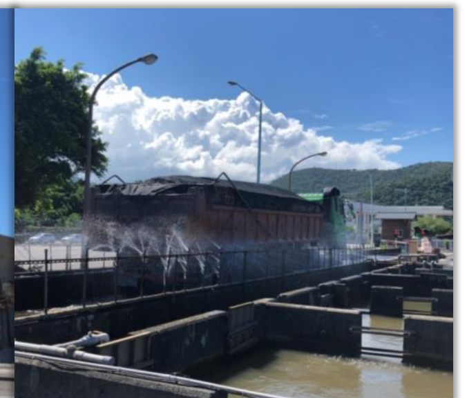
Port of Suao combines vehicle scales with car washing stations to make pollution control more efficient and effective.
