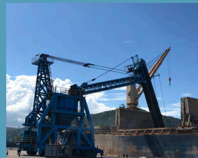
Port of Suao uses automatic coal unloading machine to reduce one of its main air pollution sources.
